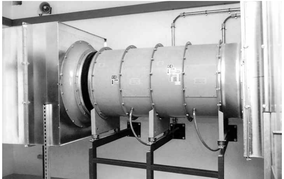
Type BVZAXN 12/56/650 two-stage axial-flow garage smoke exhaust fan for 400°C - 120 minutes (tested according to EN 12101, Part 3) in a multi-storey car park at Stuttgart airport
